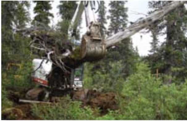
An excavator is a good tool for grubbing and slash disposal because it can pluck stumps, scatter material without damaging other vegetation, and strategically place material to help control use.
