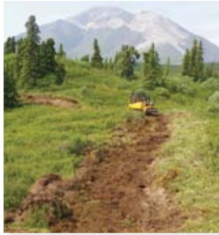
This trail has been cleared and grubbed. Rough access is being pioneered in.
