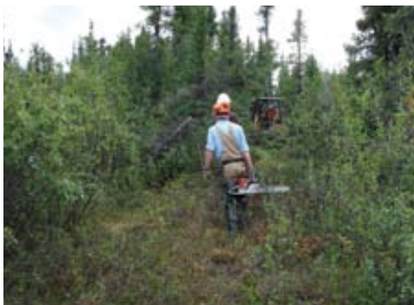
Working ahead of the trail dozer, this crew has cleared the trees and heavy brush.
