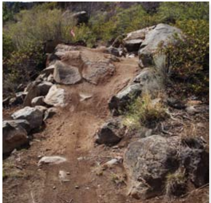
This was manufactured to provide a choice of at least three approach lines.
