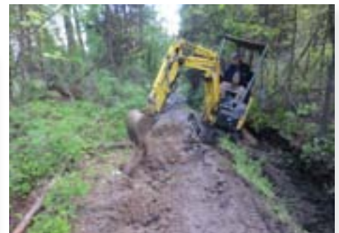
A ditch is being cut along this trail to drain the trail tread and intercept water seeping out of the inside bank. Note that the excavated material is being used to raise the elevation of the trail tread.
