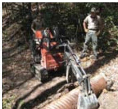
Removing culverts reduces maintenance, restores natural hydrology, provides a dip for trail drainage, and improves aesthetics.
