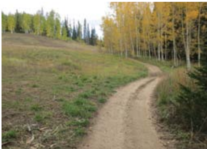
Good trail location. This trail follows the edge of the vegetative change and it curves with the natural curve of the tree line. Had the trail gone through the middle of the meadow, it would not fit our perception of “natural.”
