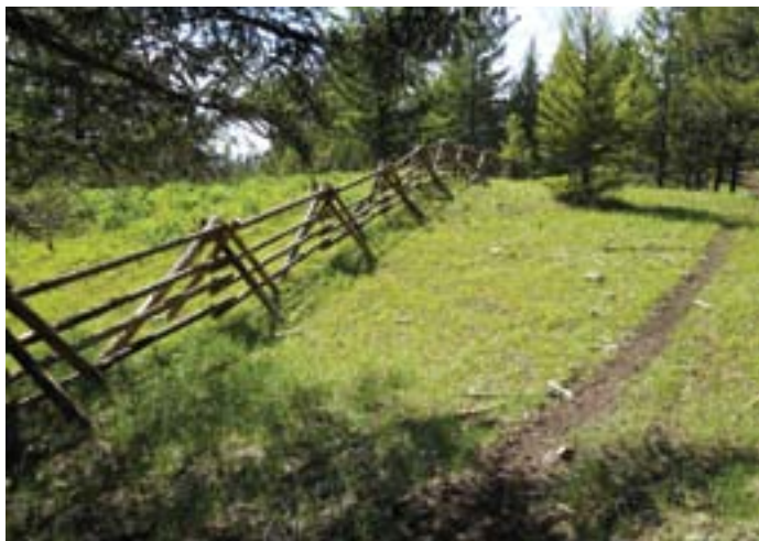
This Russell fence provides a scenic edge for this trail. Though artificial, the edge fits the landscape and enhances the rider experience.
