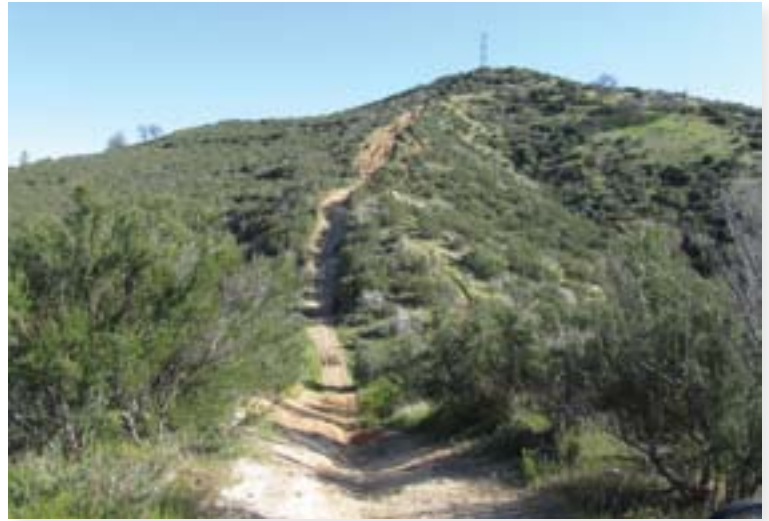
This ridgeline trail bisects the landscape and doesn't fit the natural shapes and contours. It doesn't vary the viewshed of the rider and it's boring because it is so predictable. Ridgetop trails are fall line trails and generally don't drain well. This trail definitely fits into the category of too long and too steep.
