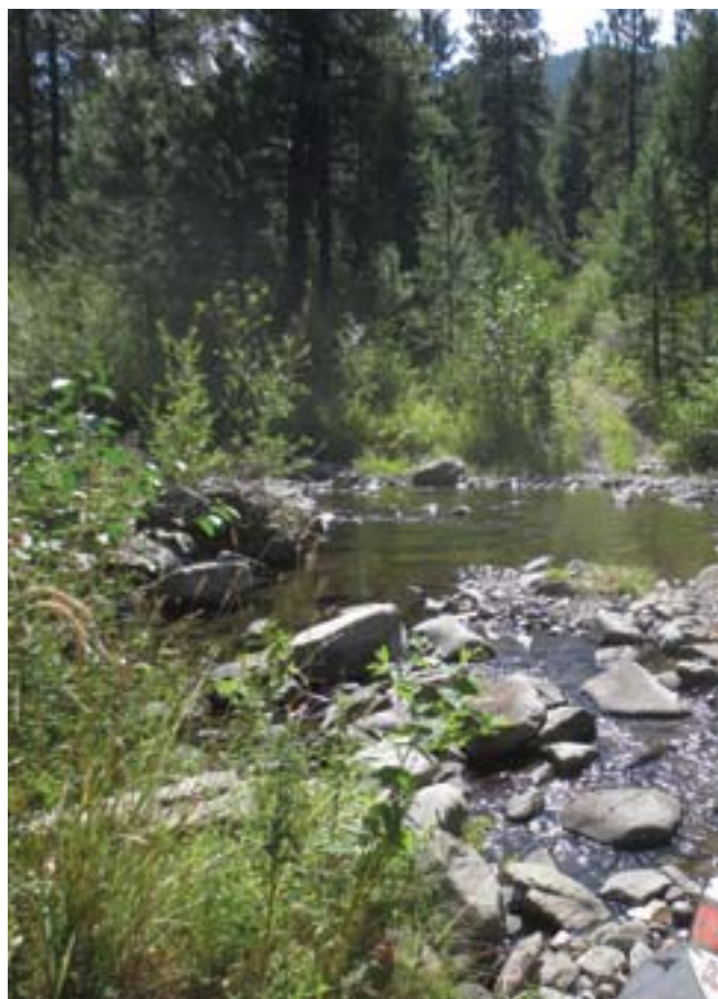
This crossing has relatively flat approaches, but large boulders at the approach and in the creek could cause potential impacts.
