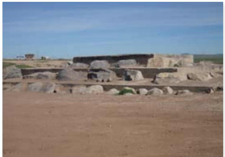
The cement and rock structure has different levels of difficulty on each side to offer a 4WD rock crawl to various skill levels. It was simple to build and will last a long time.
