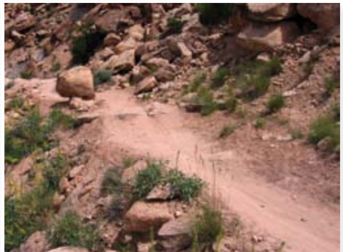
The same installation after it has settled in. No longer a smooth approach, the rock has become a challenge feature which is okay if that is consistent with the TMO.
