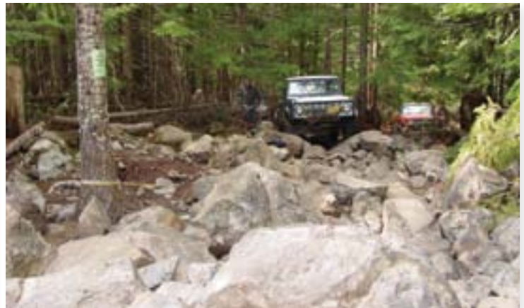
A nearby highway project needed a waste area for rock and an OHV manager needed more 4WD challenge opportunities. A win-win deal was struck and a U-shaped rock garden was created. While only about 300 feet long, it can provide hours of seat time. Note the strategically placed winch tree(s) and signs for straps required.
