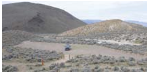
This one way in, one way out, pull-through design has great flow. The angle of the sides "tells" the drivers the angle to park and there is a sign at the entrance to park in the center. There is now a kiosk at the trail access point where three trails take off.
