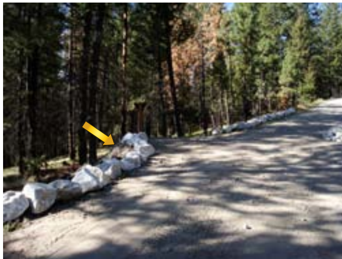
This approach has been built up with fill (arrow) so there is a level platform to stop, look, and start. Note the Yield sign. This is a functional and professional looking road crossing. It costs more, but public safety is worth the cost.
