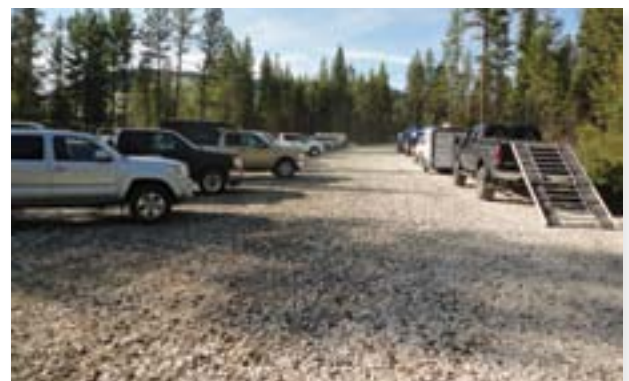
This pull through lot is 110' wide. When there is an event, there is room to park along both shoulders and vehicles without trailers can double park in the center.
