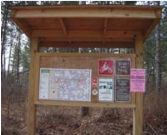
This kiosk at a trailhead contains a laminated map of the trails, a quick reference of which vehicles are allowed on the trails, and other information the riders should know, all covered with a polycarbonate shield. The seasonal closure is clearly evident. This is a good example of a good looking, well-kept kiosk.
