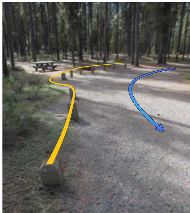
This pull-through has poor flow that can trap drivers. When pulling in from the upper end, the drivers are hugging the bollards on the left and watching the trees on the right (not shown) to make sure their trailers clear them. Then the radius of the bollards tightens up forcing the drivers to crank the wheel some more or back up. All three of the bollards in the foreground have been hit.
