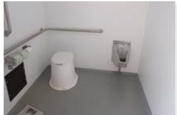
Porta-potties have had a urinal and a riser for years. Including one in the vault toilet makes sense, but there is also more to clean.
