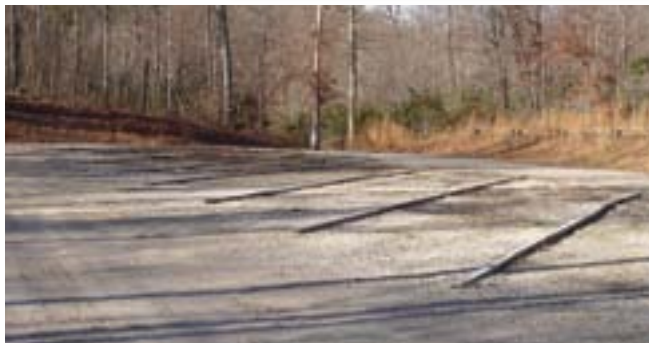
These treated timber parking delineators are expensive, inhibit parking lot maintenance, and don't work well to organize the parking. People will be driving over them and tripping over them. A Park in Center sign would help. The angle of the parking should be determined by the angle to the parking lot entrance. If it isn't, one row of timbers would be sufficient to guide the first vehicle.
