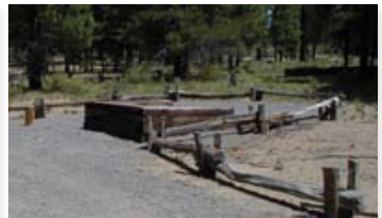
This was built as a volunteer work party project using old railroad ties. It's not fancy, but it works. The barriers prevent kids from using it as a jump.
