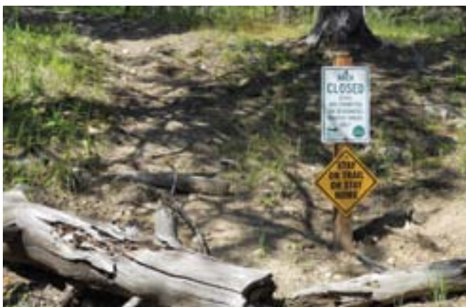
This is a good example of closure tools; ripping, blocking, seeding, and signing. The Stay on Trail or Stay Home sign is a great sign, but it sends a confusing message here. Is the rider supposed to stay on the open trail or the closed trail?
