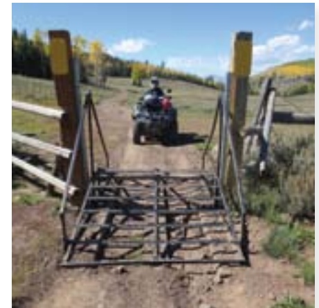
This narrow cattleguard is being used for both range management and entrance management.
