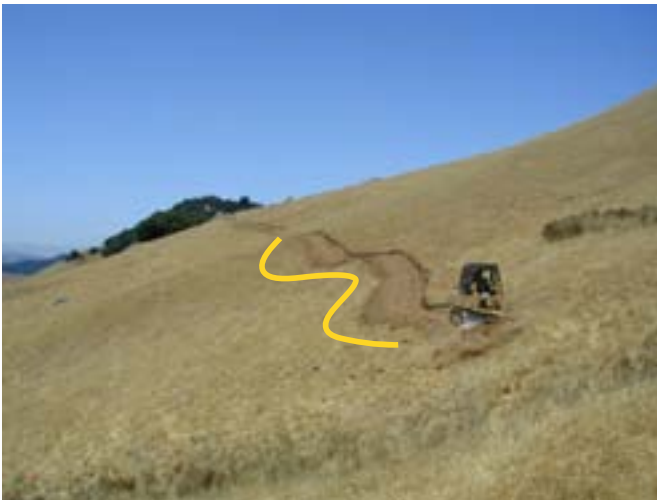
Locating a fun, sustainable, and visually unobtrusive trail on an open landscape can be challenging. Note the undulating W shape of this location. If nothing else, this trail will drain well.
