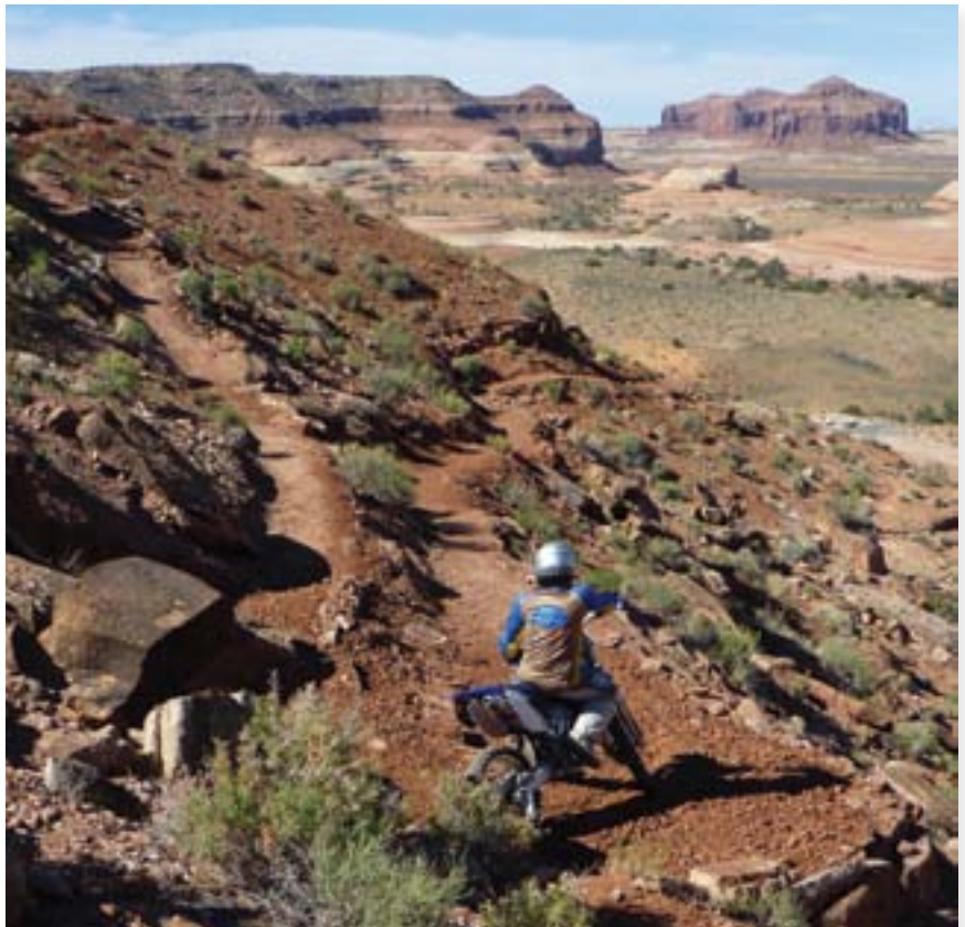
A nicely-designed switchback. Notice how the grade of the upper approach flattens off before the landing. This adds significantly to the rideability of the structure. The landing is long and wide to allow room for a smooth turn on a circular curve.
