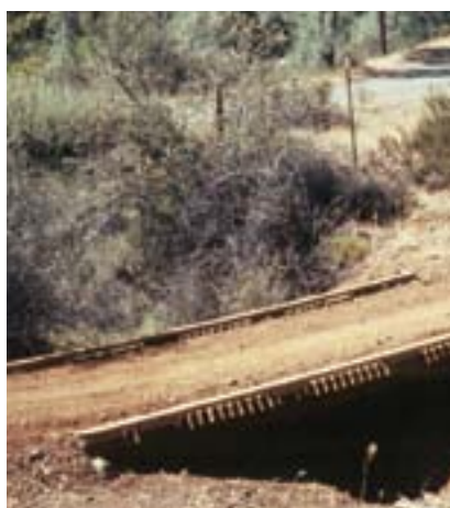
This bridge is in the bottom of a grade sag so water and sediment collect and drain in the middle of the bridge. When this creek is flowing, sediment will be delivered directly into the water. If this was a perennial, fish-bearing stream, this bridge site would not be acceptable.
