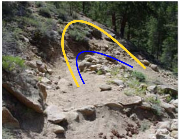
This structure has a nice circular curve, but no flattened approaches. Note the drain above and there's one below also which is good. It may have been better for drainage and rideability to use the top of the exposed rock as a flat area for the lower approach and part of the landing.
