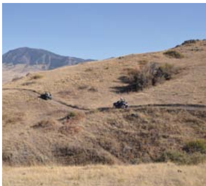
Even in an open landscape, this trail flows with the terrain, drains with the terrain, and has minimal impact on the terrain.
