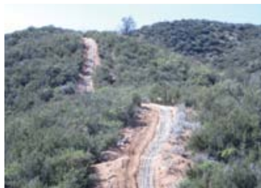
Adding trail hardening to a long, straight, fall line trail. Is it a fix or a solution?
