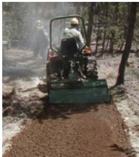
Bentonite clay being rototilled into non-cohesive pumice soil.
