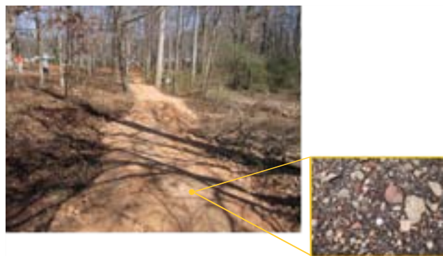
This hardening installation is another recycling project. A brick and concrete high school was being torn down and was headed for the landfill, but a heads-up project planner thought to grind it up and try it for trail hardening. The material was free, it worked, and it set up like concrete due to a good mix of particle sizes. This was a win-win for the project, the community, and the environment.
