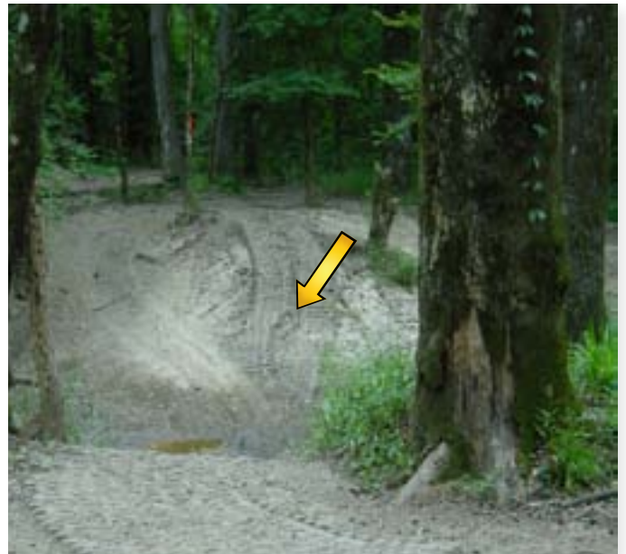
No containment, no protection for any of the edges, and uneven surfaces. Note the settling that has occurred (arrow) between the two rows of blocks. Given a choice, which there is, any rider would avoid this.
