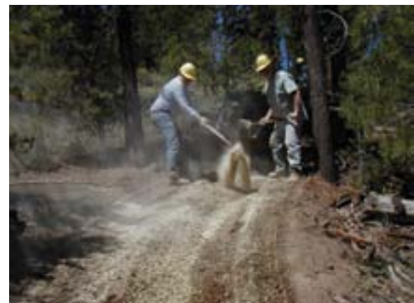
When the spreader box plugged up, the eyeball measuring and hand distribution methods were used.
