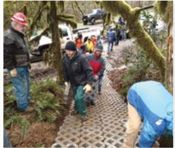
Having an army of volunteers certainly helps with a trail hardening project.
