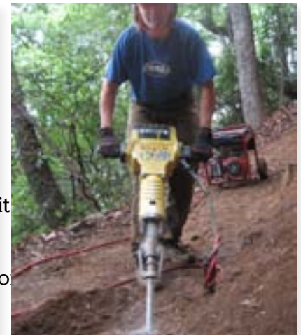
Pneumatic rock splitters clear away stubborn rocks in the tread.
