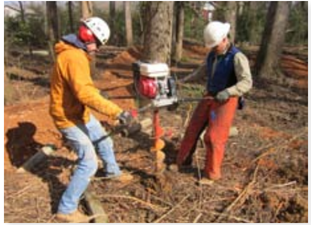
Gas powered augers save time and hands for sign post or fence installation.
