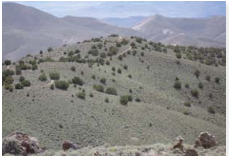
This is a much better example of how a trail that follows the ridgeline can harmonize with the landscape. The serpentine alignment switches from one side of the ridge to the other. This creates drainage and varies the rider viewshed. Very little of it is on the actual ridgetop except for the last rise. When the rider tops that crest, he is presented with a panoramic and totally WOW view of several mountain ranges.
