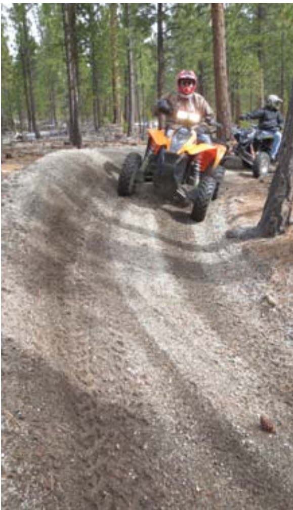
Superelevated curves can reduce the effects of displacement. On a curve like this, any soil particles that are displaced will roll back down into the tread.
