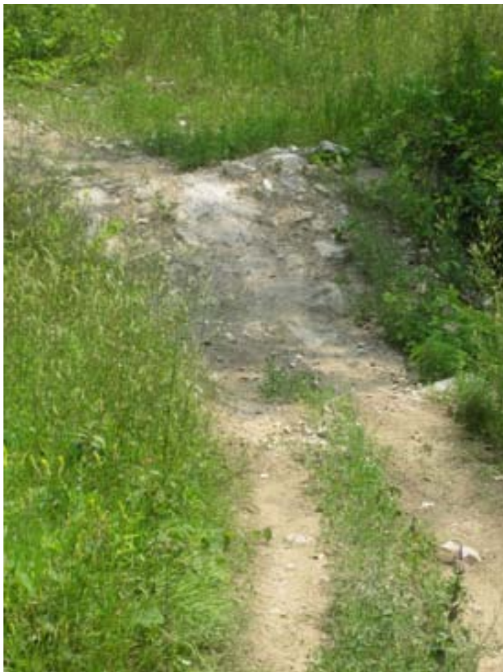
This rock outcropping was used as a pivot point for a curve in the trail. The rocks help stabilize the soil and increase the variety in the trail.
