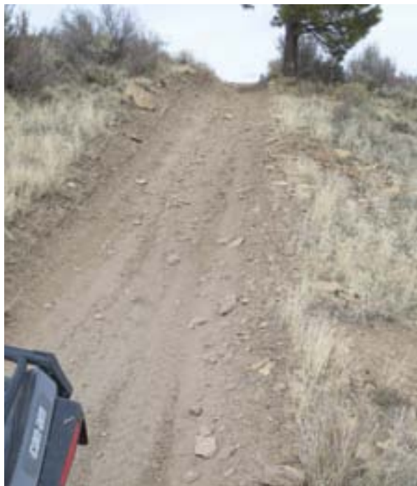
The high rock content on this grade has made it durable. The grade is steep (25%) but short (50'). In spite of a dramatic increase in use, this slope has changed little in 15 years of monitoring.
