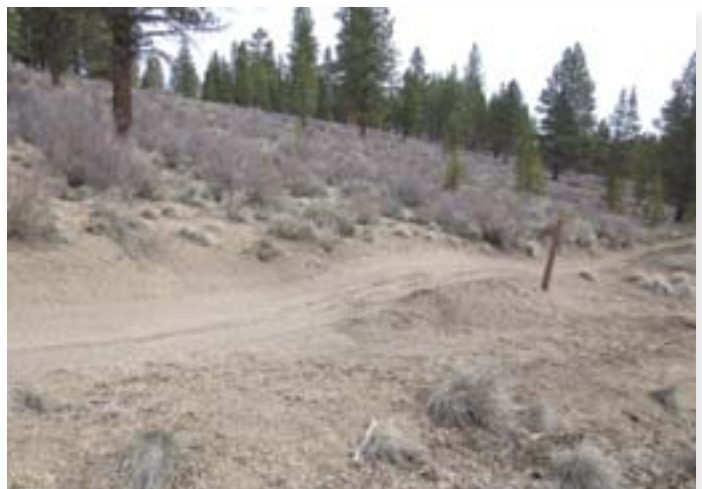
Though this dip rides nicely, it wasn't constructed with enough elevation difference from the sag to the crest. Due to the soft, non-cohesive soils, displacement from a few motorcycles has already created a rut deep enough for the rolling dip to fail.
