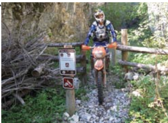
This is a good example of an entrance management installation: well-placed barriers backed up with good signing. The 4Es at work.
