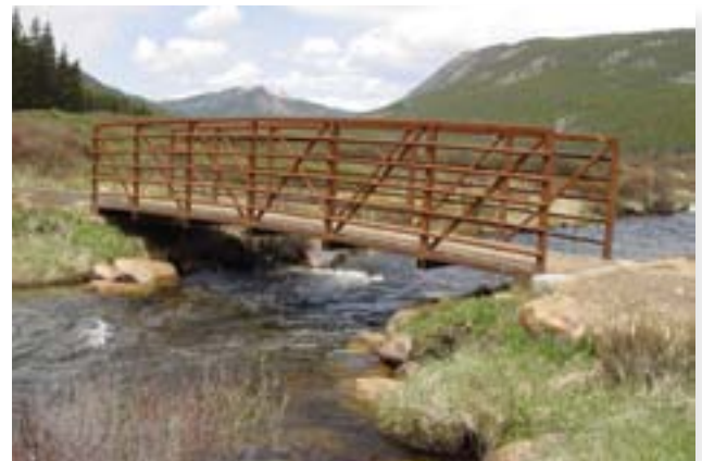
This prefabricated steel bridge is durable and has a natural appearance in this open setting.
