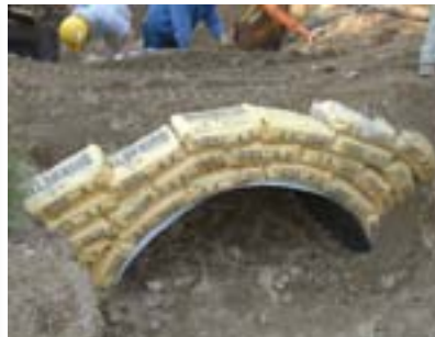
When rock is not available or when extra support or protection is needed, bags of pre-mix concrete will make a solid headwall. They will absorb moisture over time and solidify into a concrete block wall. Do not use sandbags since the bags will eventually rot and your structure will disintegrate.
