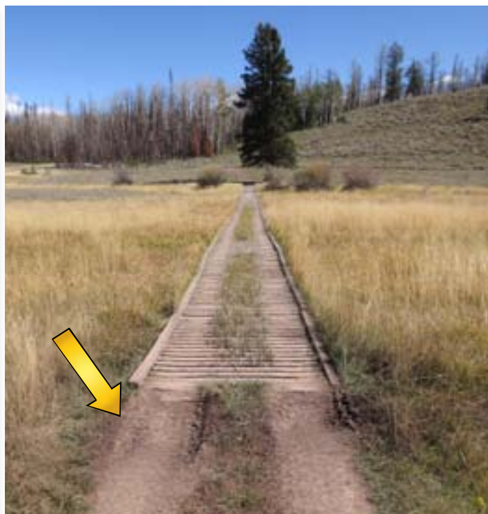
One of the oldest trail structures, puncheons can be beautiful, functional, and fun to ride. Note the muddy spots where the structures end too soon (arrows). These should be filled with rock or hardened with a geosynthetic and a rock cap.
