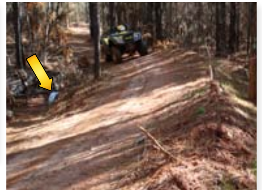
This heavily superelevated curve is a blast to ride, but water runs to the inside, gets trapped, and ponds up. The solution? Add a culvert.
