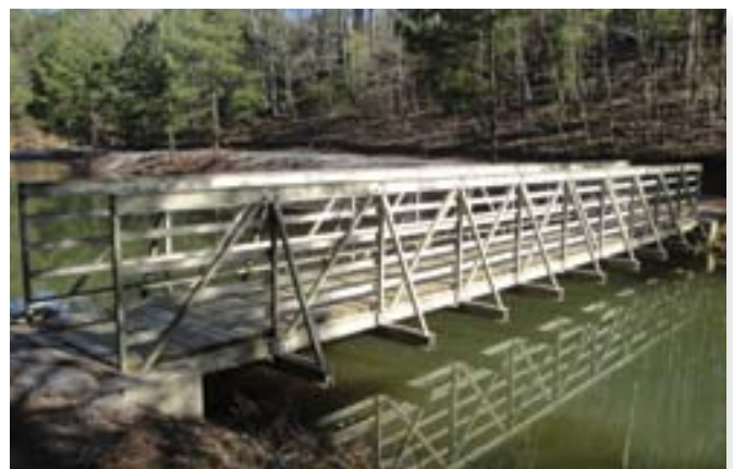
With transport and assembly advantages, a fiberglass pony truss bridge can work well in a variety of settings.
