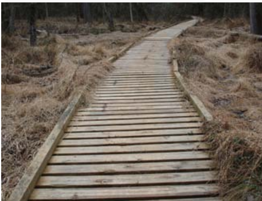
One of the oldest trail structures, puncheons can be beautiful, functional, and fun to ride. Note the muddy spots where the structures end too soon (arrows). These should be filled with rock or hardened with a geosynthetic and a rock cap.
