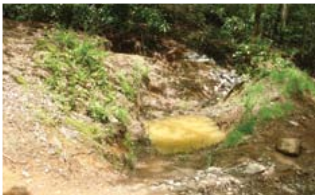
Due to the flat terrain, this rolling dip has little elevation difference between the sag and the crest. The lead-off ditch also has a flat gradient and it is almost full of sediment. Notice how the water is flowing past the entrance to the ditch and is almost breaching the rolling dip (arrow). If maintenance isn't performed shortly, this structure will likely fail.
