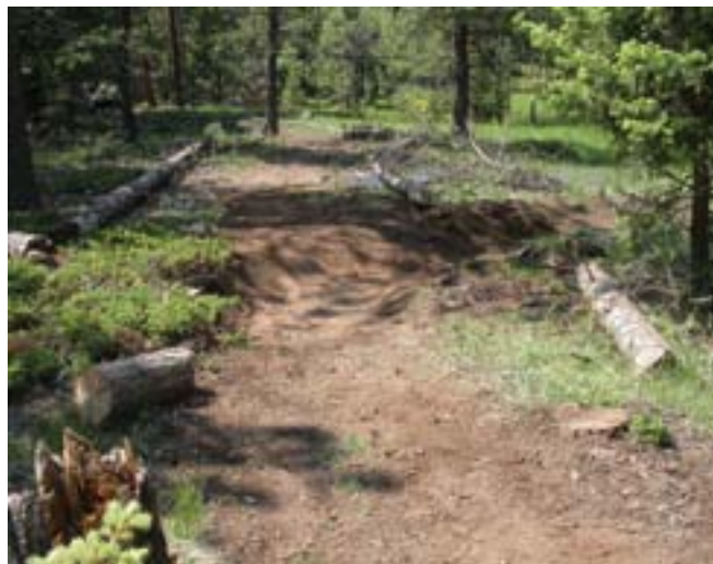
A nice lead-off ditch was constructed to drain a rolling dip, but as riders' eyes scan this area, it is difficult to determine a ditch or a trail going off to the right. A millisecond of uncertainty can draw a rider into the ditch. To avoid this, it is a good practice to place a small log across the ditch entrance so it spans the ditch without blocking the flow of water.
