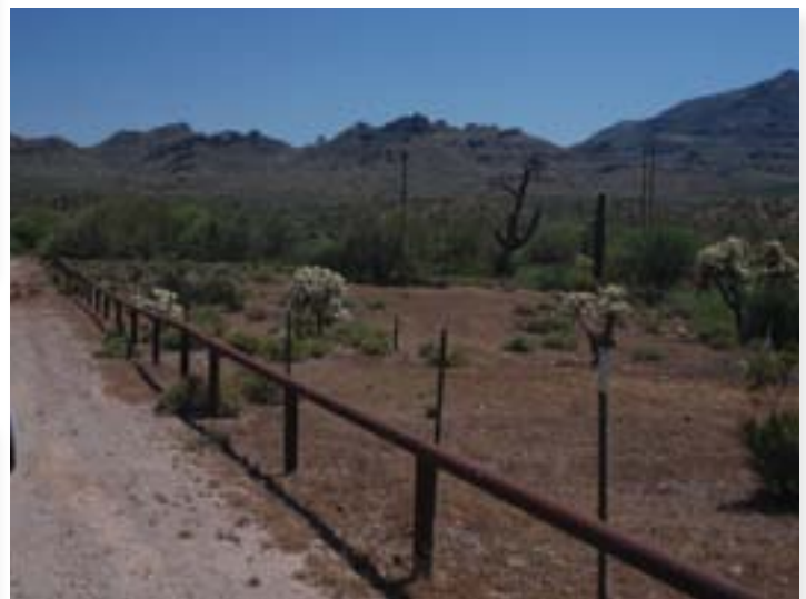
With no other materials readily available and in an area prone to vandalism, these pipe barriers are a good choice.
