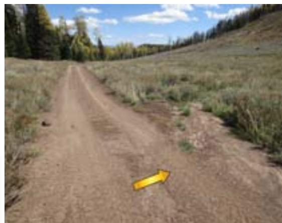
Due to the flat terrain, this rolling dip has little elevation difference between the sag and the crest. The lead-off ditch also has a flat gradient and it is almost full of sediment. Notice how the water is flowing past the entrance to the ditch and is almost breaching the rolling dip (arrow). If maintenance isn't performed shortly, this structure will likely fail.
