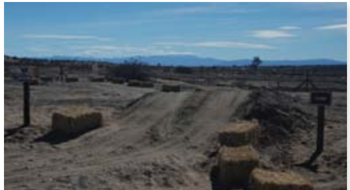
Hay or straw bales can make good barriers to control and direct the use. Their portability makes them good for short term uses like trail closures. Bales may need to be certified as weed-free.
