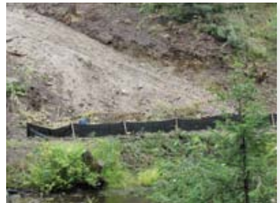
Silt fence was installed at the base of this fireline to protect runoff and sediment from entering this sensitive stream. It often comes pre-attached to wooden stakes, but they will not last as long as metal T-posts.
